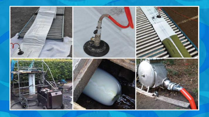
All materials used are WRC approved and are installed under the water industry specification for cured in place pipes (CIPP). Our engineers are fully trained and certificated in installation and the latest health and safety methods and are CSCS and Confined SpaceTrained.
