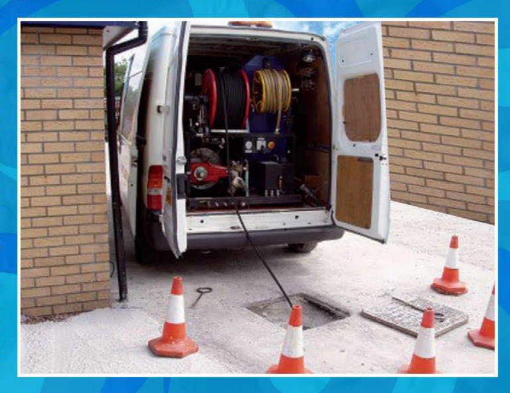
In the case of storm water drains, where high levels of sand can accumulate over a number of years, the use of water jetting is ideal for cleaning as it enables the sand to be removed after being dragged back behind the water jetting nozzle as the nozzle is brought back to the access point.
